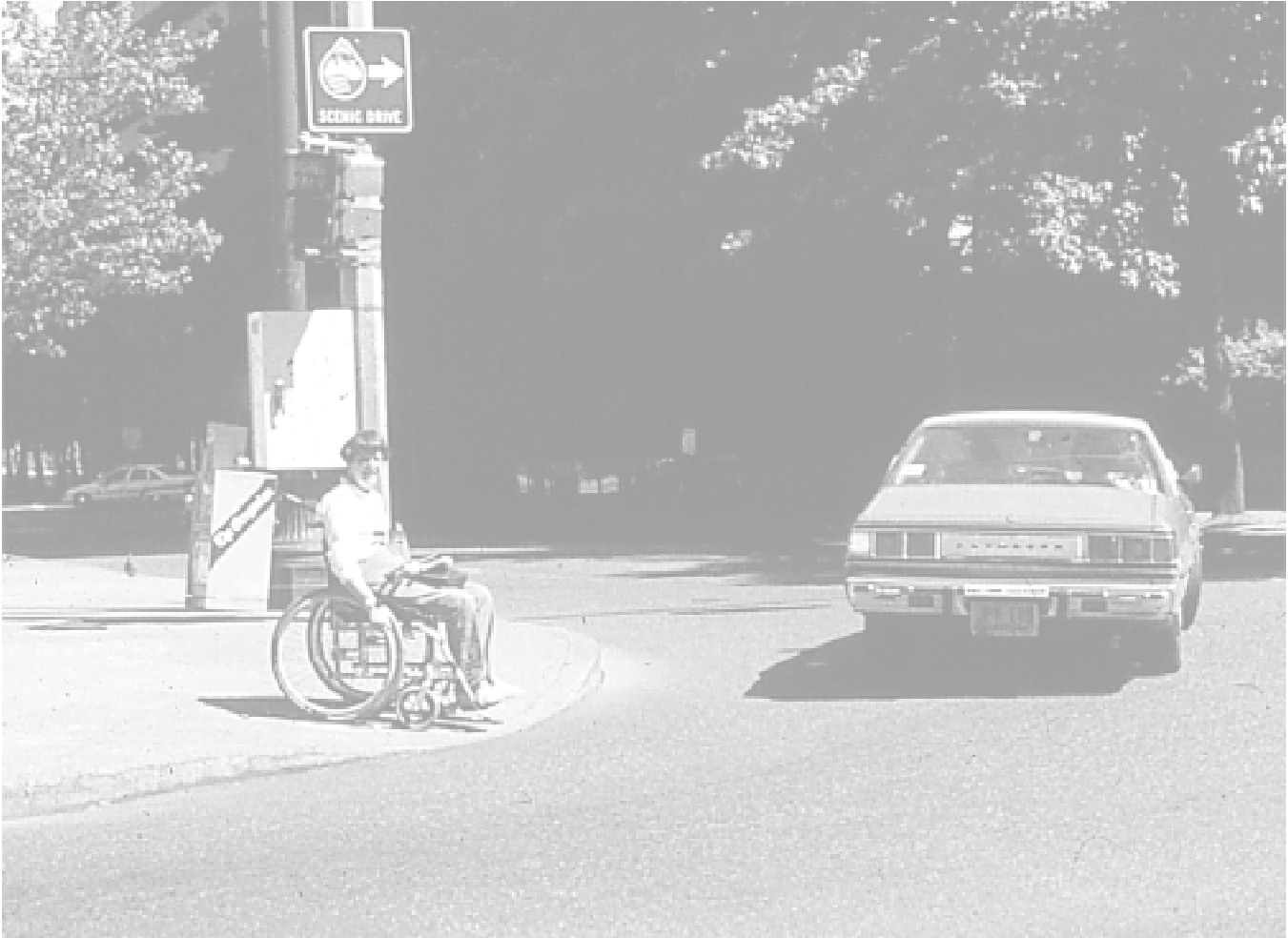
Curb ramps at corners are an important element of an accessible pedestrian network.
