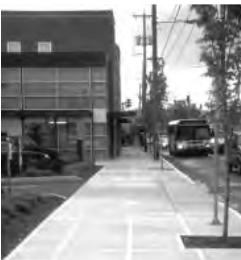
New sidewalk constructed as part of an infill redevelopment project.
