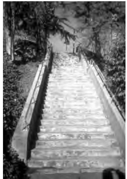
Numerous public stairs are found in Portland's West Hills.
